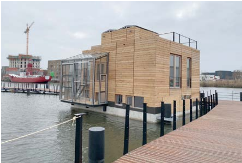
One of the first houses to be anchored. © Fraunhofer
