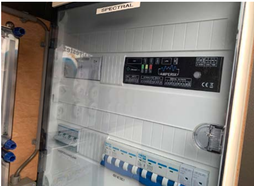
The Fraunhofer ITWM's energy management system goes by the name of Amperix®; myPowerGrid is a platform for microgrids and energy communities. © Fraunhofer ITWM
