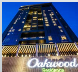
OAKWOOD RESIDENCE KAPIL HYDERABAD
